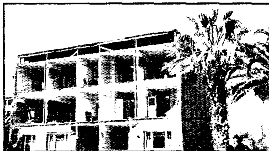
W6EQW HAD TWO MESSAGES FOR PEOPLE HERE BUT HAD TO DELIVER THEM AT "MISSING PERSONS BUREAU"
